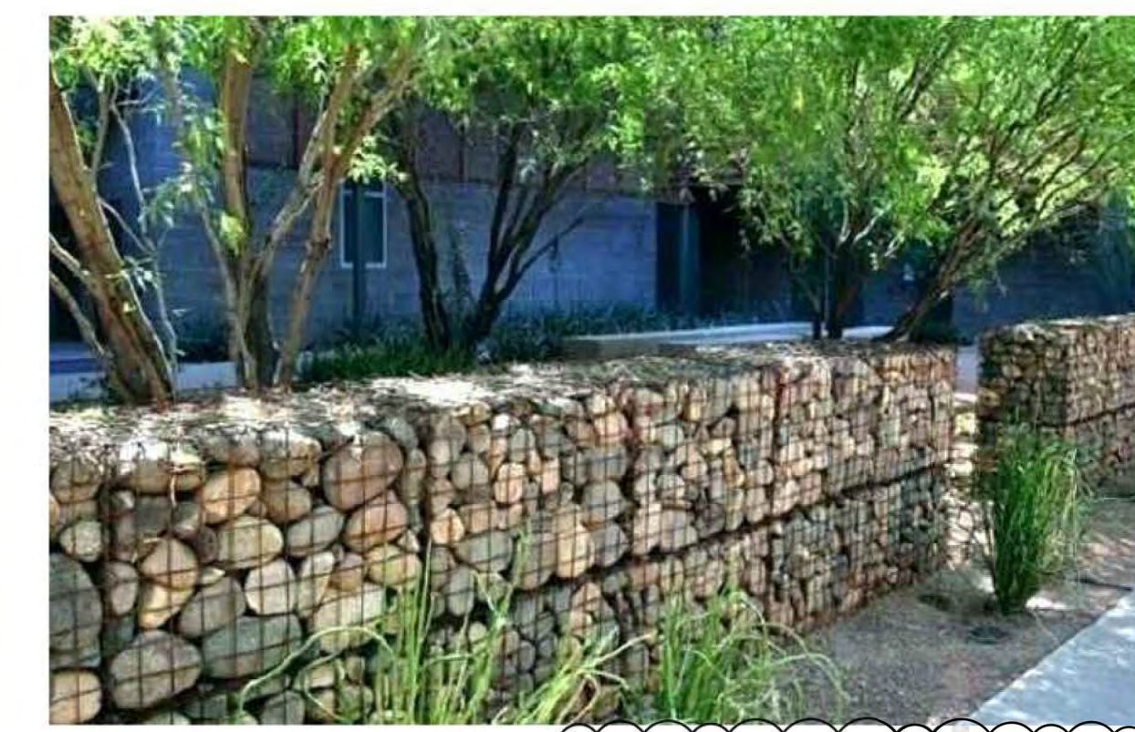
4' Gabion wall See Detail on Sheet A-10
